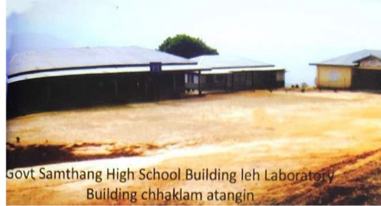
Govt. Samthang H/S building & Laboratory building
