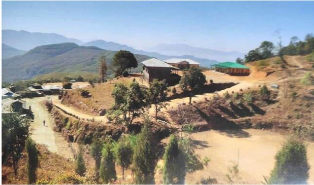
Samthang H/S Before
